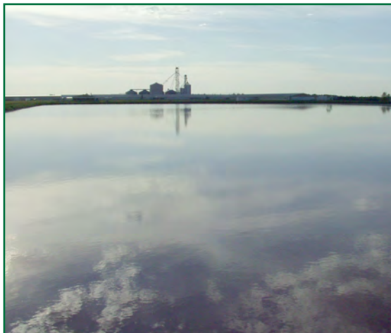
15 Million Gallon Lagoon - SD
